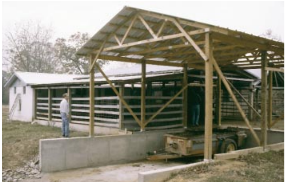
Premilk holding area with attached manure dry stack.
