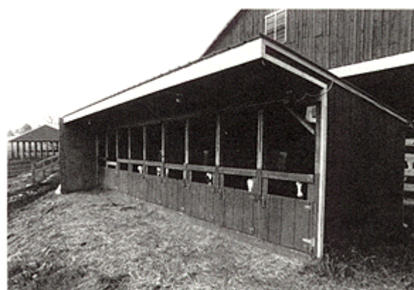
Calf-hutch type structure in a building with three of its sides enclosed.
