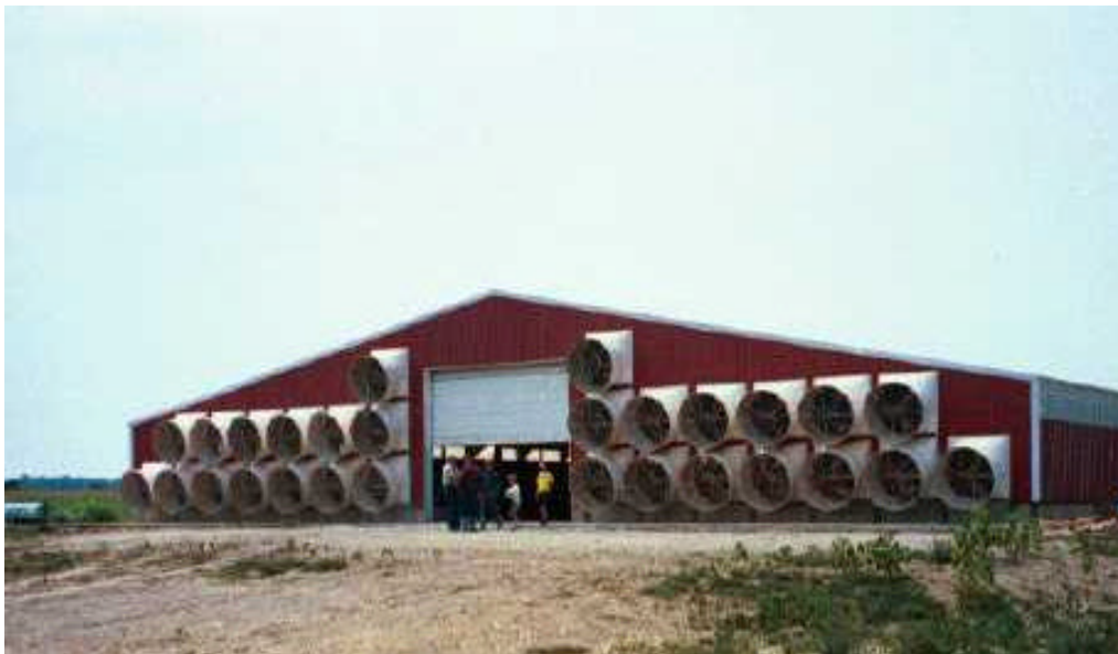
Figure 1. Tunnel fans positioned on endwall of a tunnel-ventilated 6-row freestall barn.
