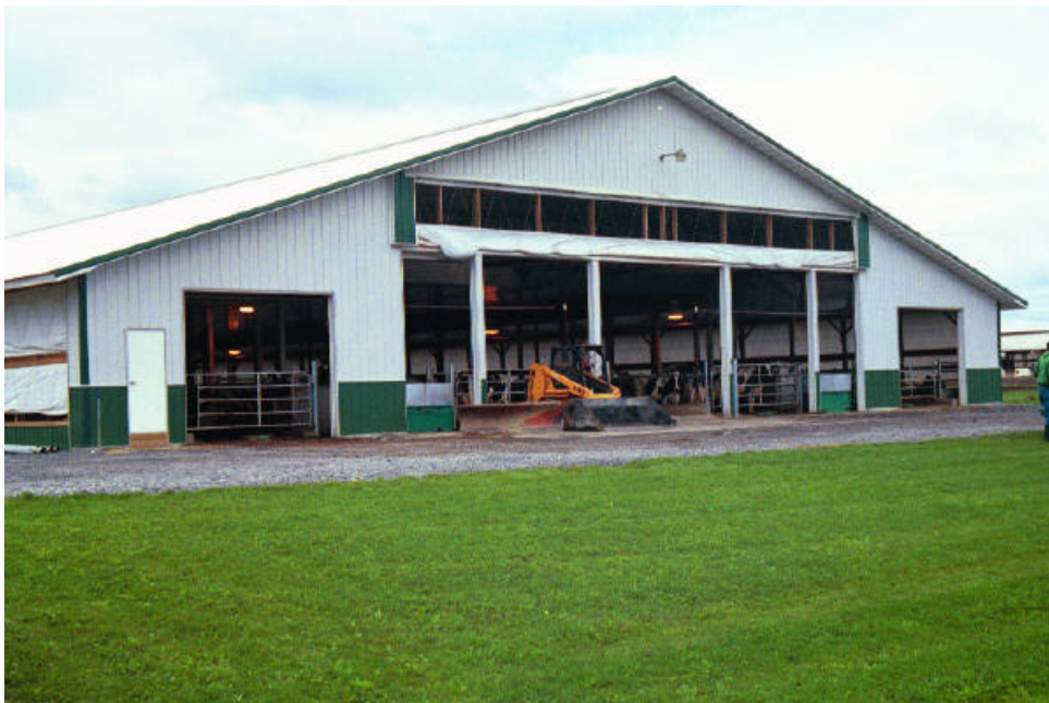
Figure 2. Inlet for a tunnel-ventilated 6-row freestall barn.
