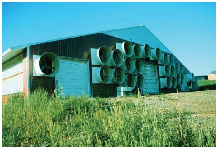
Figure 7. Tunnel ventilation in free stall barns requires lots of fan power
