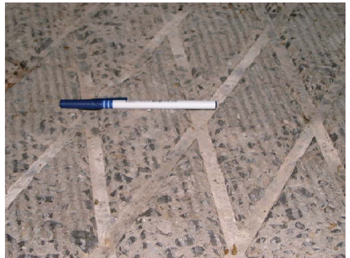
Figure 11. Surface milling to improve traction
