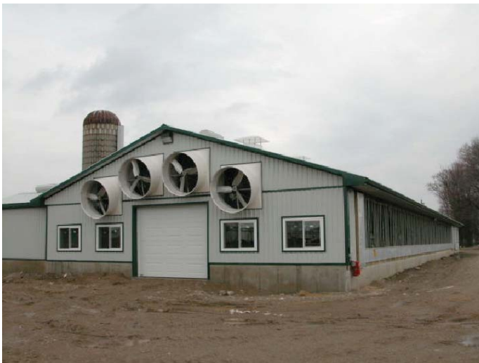
Figure 6. Tunnel ventilation in a tie stall barn
