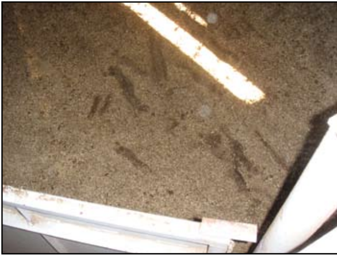
Photo 7. Worn cement results in slips on the dock.
