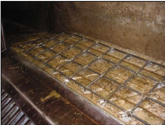
Photo 14. Welded grating on stun box floor.
