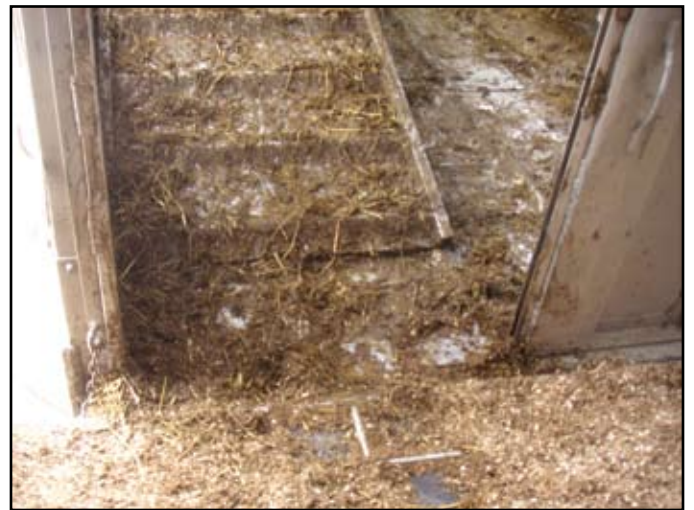
Photo 6. Steel grating on landing to improve footing.
